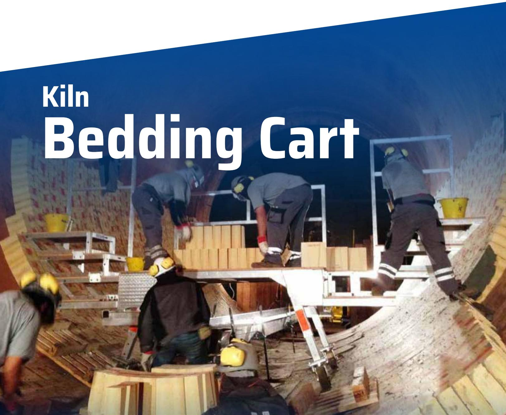
**Speed up bedding out larger kilns** while providing a safe, ergonomic working deck with stairs for higher brick placement.
